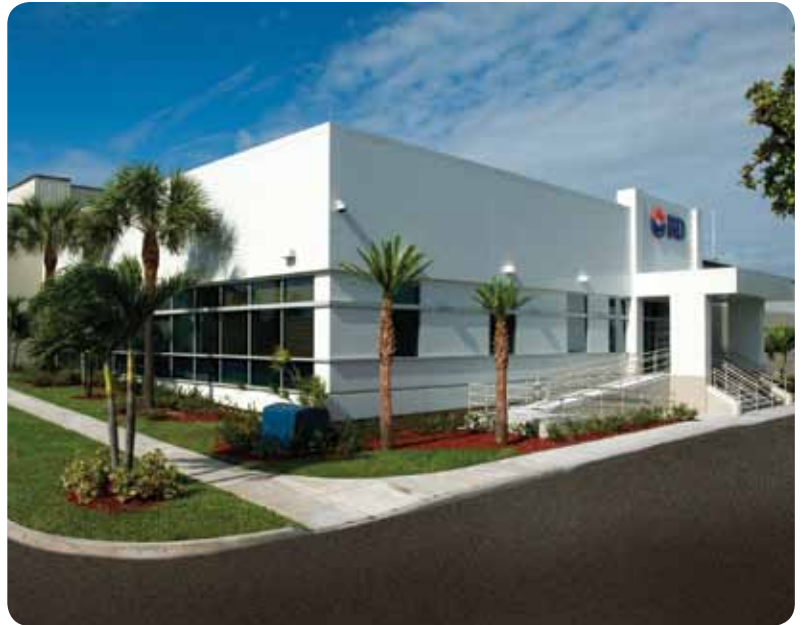
The first stand-alone, dedicated, animal free, antibiotic free (AF2™) production facility for the cGMP production of high performance cell culture media and supplements.
